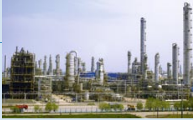
SAMSON supplied around 1,800 control valves to the new BASF site in Nanjing, China, their third largest site worldwide.
