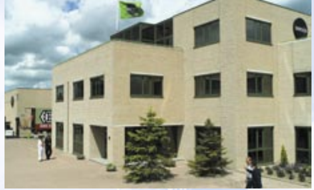
The building of SAMSON REGELTECHNIEK B.V. in Zoetermeer, a city situated close to The Hague, Amsterdam and Rotterdam.
