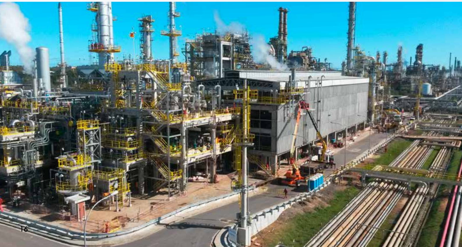
View of the Alberto Pasqualini refinery (Refap) located in Rio Grande do Sul.
