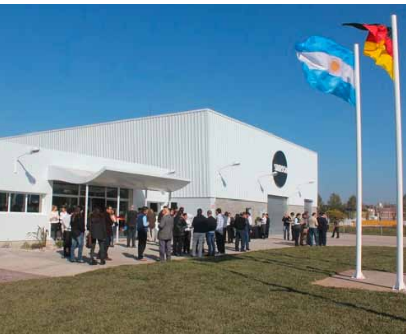
From the new building in Buenos Aires, the Argentinean subsidiary serves customers in Argentina, Uruguay and Paraguay.
