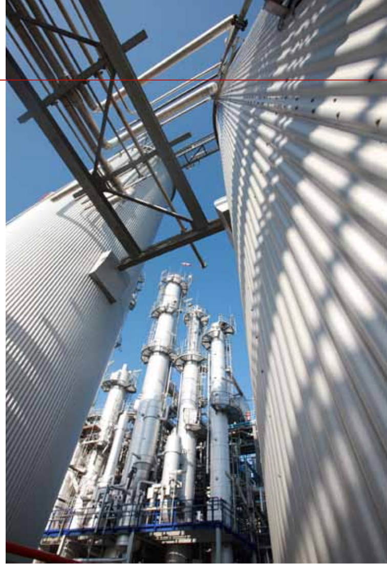
SAMSON control valves are also used at Evonik Industries, an international supplier of specialty chemicals.
