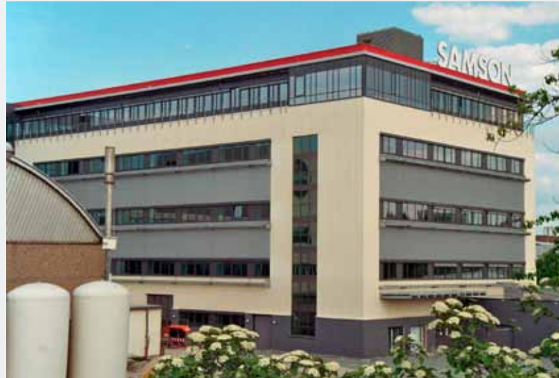
The new production hall with a floor area of 3150 m 2 and a height of 28 m is one of the largest buildings at SAMSON.
