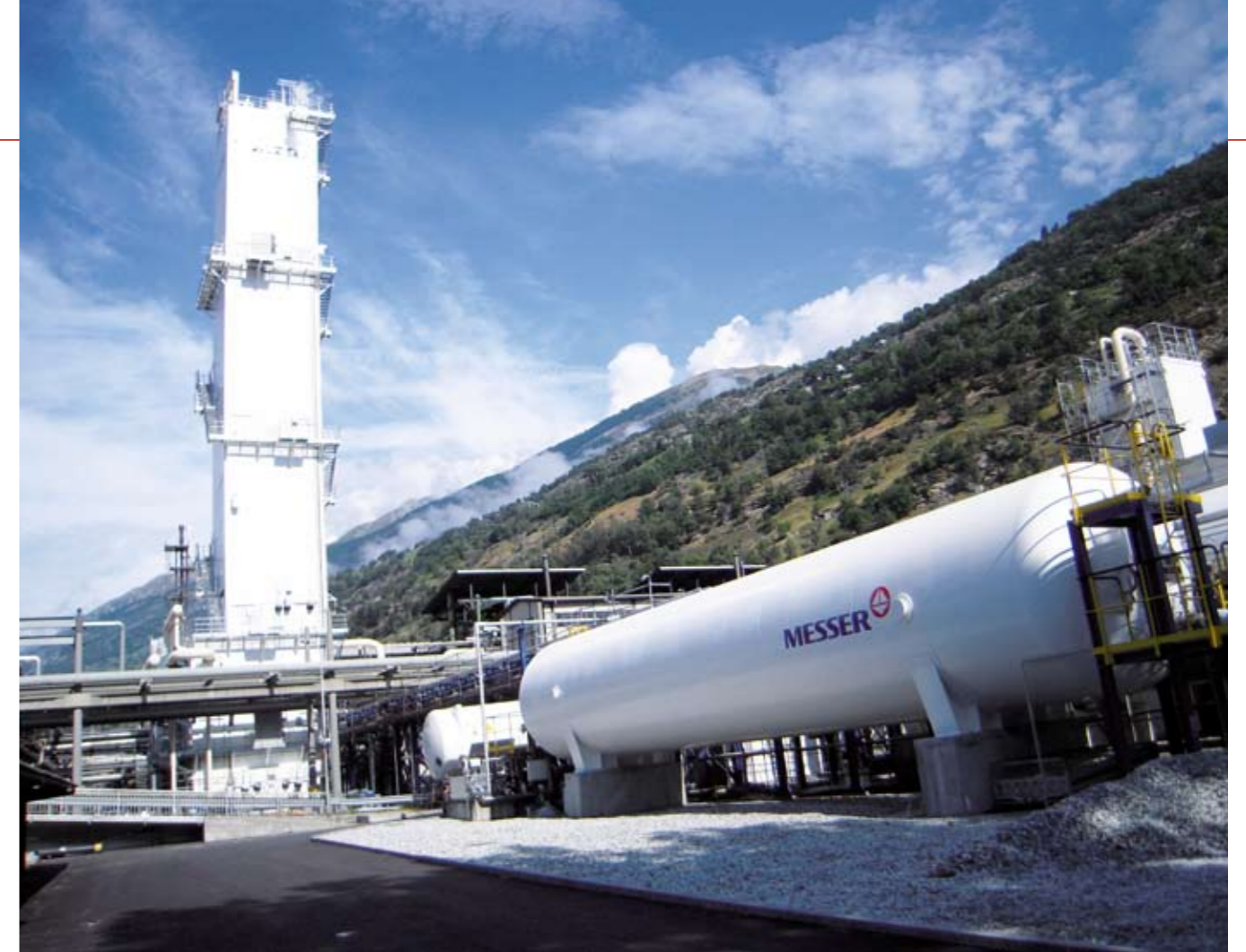
With a height of 60 m, the air separation plant on the premises of Lonza AG at Visp is the highest building in the Swiss canton of Valais. Messer invested around 20 million euro into the on-site production of industrial gases and medical-grade oxygen.
