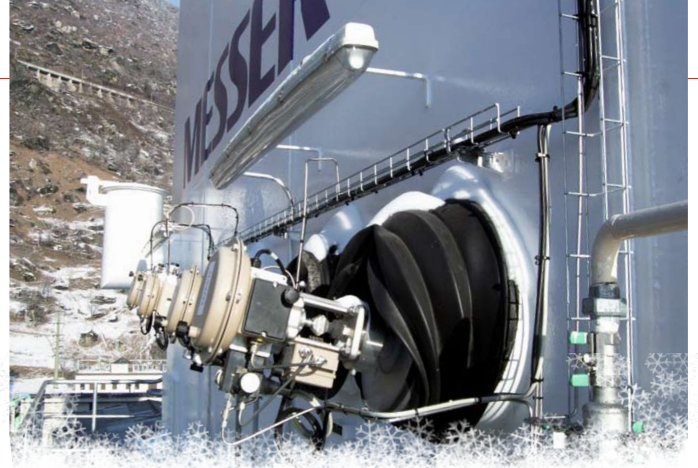
The bellows seal on SAMSON's cryogenic valves keeps the cold in the cold box and reliably prevents the outside parts from icing over.
